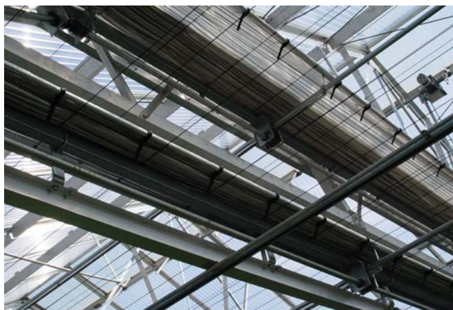
Top: Many growers are now installing dual curtains to reduce energy consumption. Bottom: Installing roll-up walls with durable drive units can offer growers a long-lasting automated solution to energy consumption.
