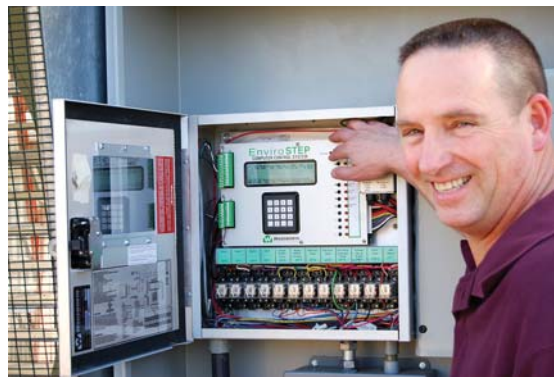
Upgraded environmental control systems offer ramping, which is a gentle transition from day to night temperature settings. (Photo: Jane Bergantz)
